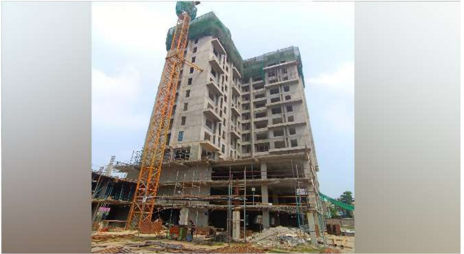
TOWER-2, 15TH FLOOR LEVEL ALUFROM AND SLAB REINFORCEMENT WORK IN PROGRESS
